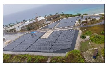
The Energy Conservation Measure (ECM) shown above includes 2,380 kWdc of solar Photovoltaic (PV) electricity generation, a 2 MW / 3 MWh lithium-ion battery Energy Storage System (ESS), and microgrid control system on the island of Meck, in the Marshall Islands. This reduces the island's dependence on diesel fuel electricity generation by an average of 55% throughout the ESPC performance period and provides energy resilience to critical missions located in the region.
